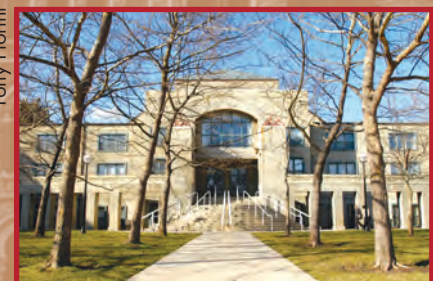
School of Architecture and Planning moves into the Edward M. Crough Center
